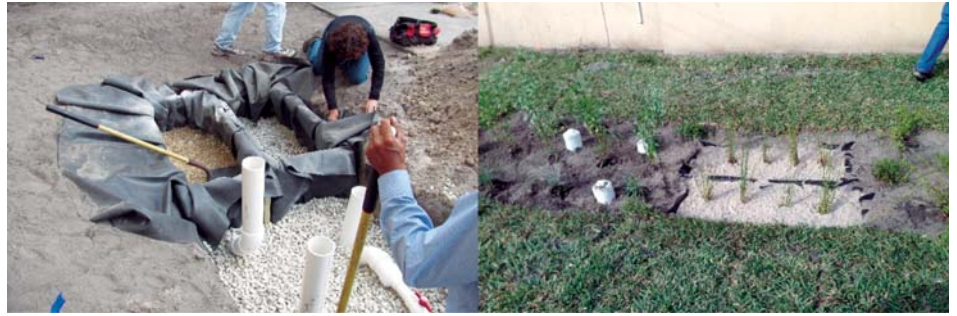
Figure 7. Installation (left) and Installed Bioretention Cells (right) at the Spotford Center
