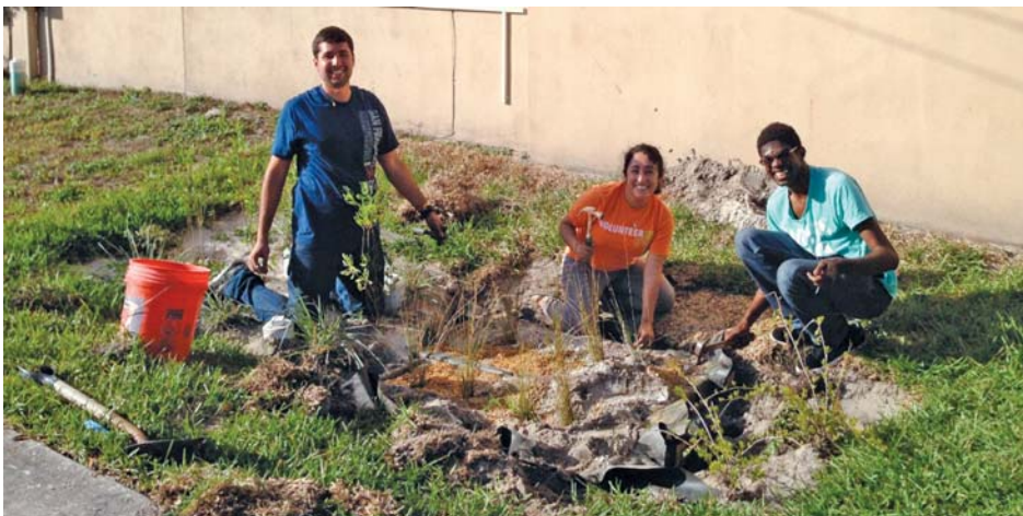
Figure 8. Rehabilitation of Geomembrane Liner and Plant Maintenance After First Winter
